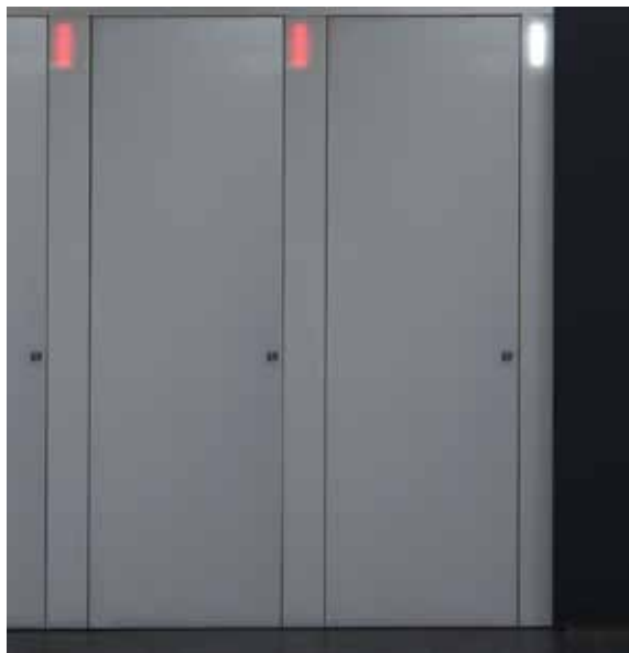
LED occupancy indicators are a higher-end solution that replace conventional lock indicators.
