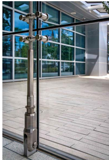
Planar Net fitting assembly
