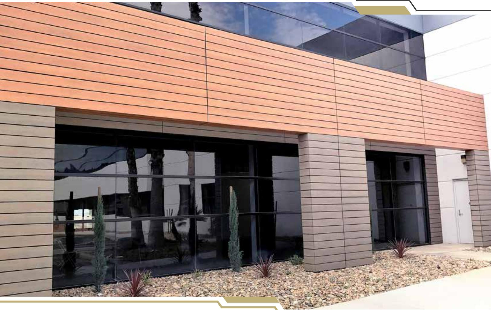
**Sizes:** 4"-24" in Height, 8',10', or 12' in Length, and 8, 10, or 13mm in Thickness
